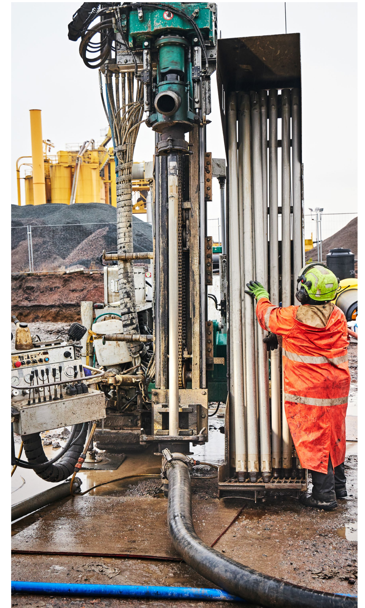
Installing ground source heat power at KOy Tuusulan Högbergintie 5, Tuusula
